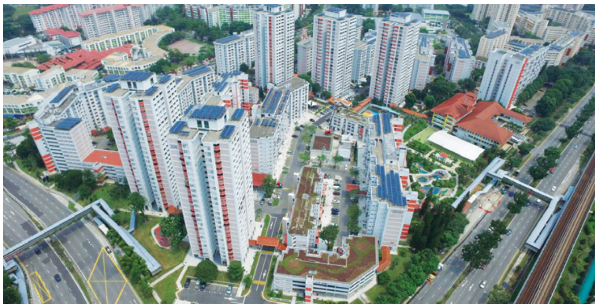
HDB Greenprint Neighbourhood at Yuhua. Solar panels and greenery are visible on the rooftops of these blocks.
