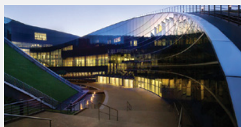
NTU's School of Art, Design and Media building has a green roof that lowers both roof and ambient temperature.
