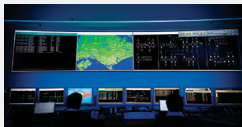
SP's SCADA (Supervisory Control and Data Acquisition) system monitors and controls the national grid, and is one of the systems that the SP Centre of Excellence will look to enhance with next-generation technologies.
