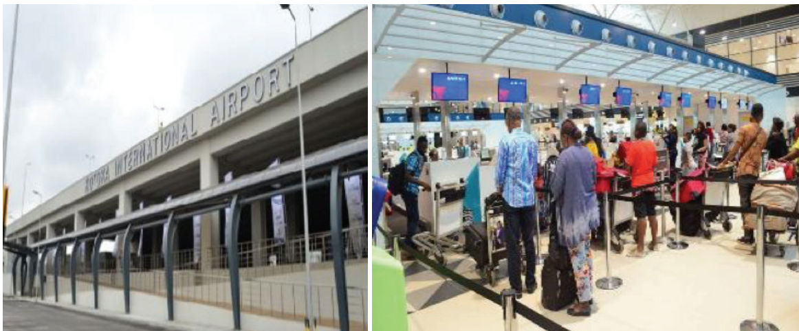
New Terminal at Kotoka International Airport, Accra
