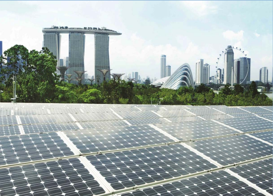
SOLAR PANELS ON ROOFTOPS
