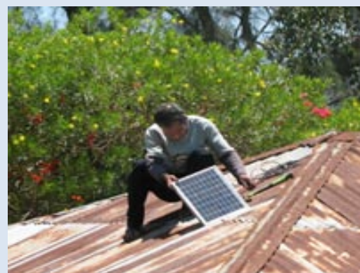
Figure 9. Solar Panel installation. Source: Alternative Technology association
