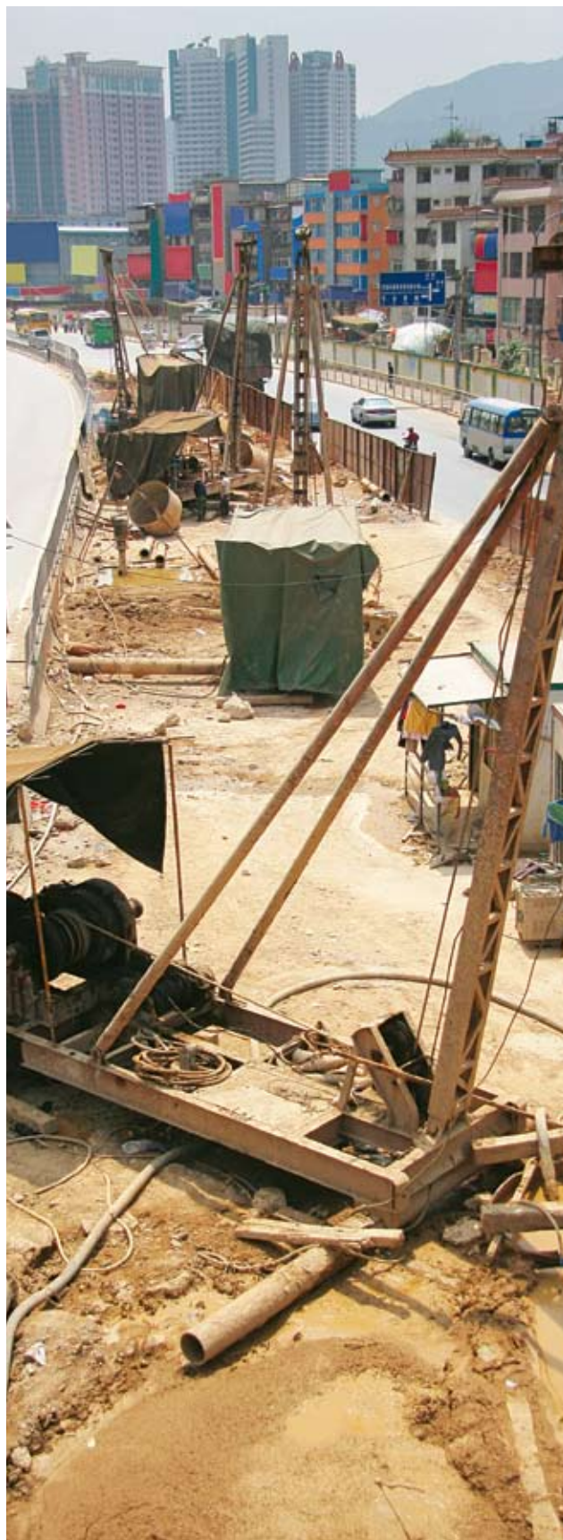
▲ Construction cranes doing ground work for a light rail system in Shenzhen, a special economic zone in China.
