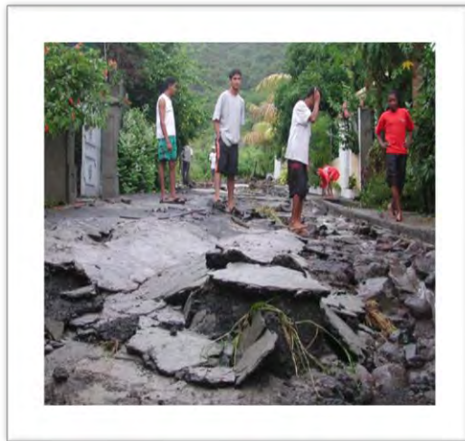
Road damaged due to torrential rains
