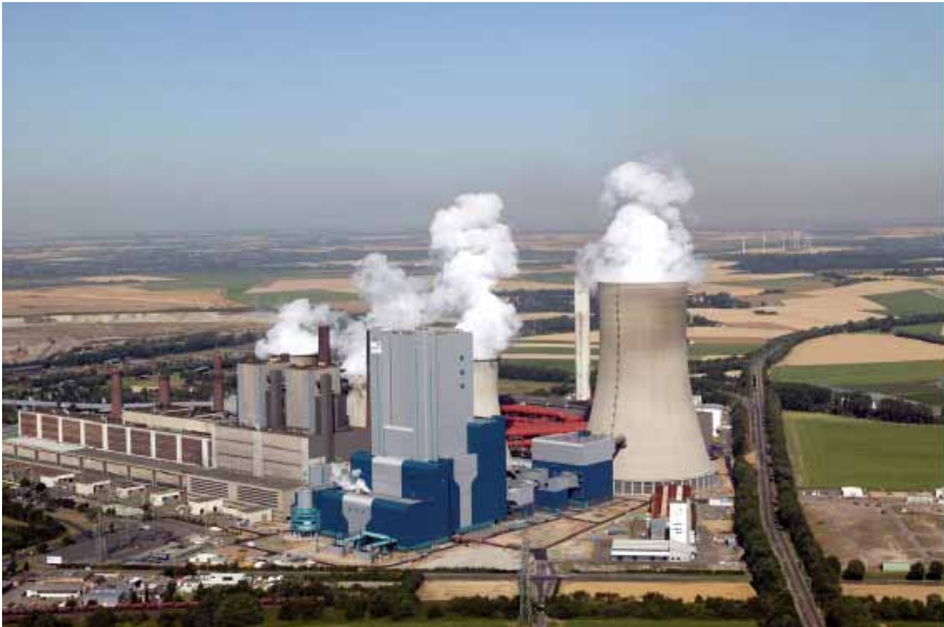
Neideraussem Lignite-fired Power Plant, 965 MWe (net), 43.3% (HHV)
