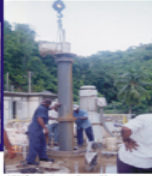
NWC workmen installing pump
