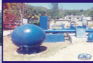
Rehabilitated pumping station
