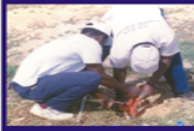
NWC workmen installing meter
