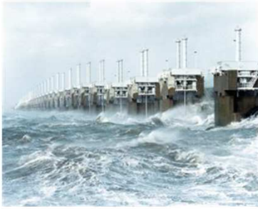
Safety, protection against flooding
