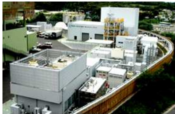
The New Energy Plant at EXPO 2005
