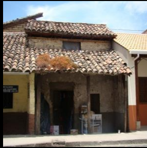
Buildings in bad condition
