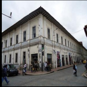
Buildings in regular condition
