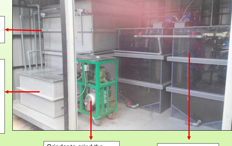
Grinder to grind the food waste – faster the digestion process
