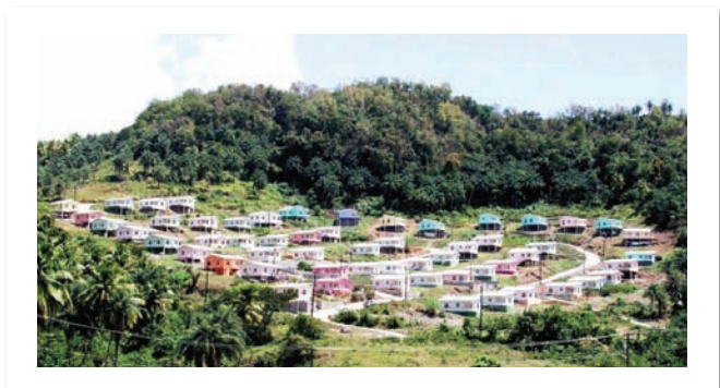
Photo 5.5: Low Income Housing Project, Peter's Hope
