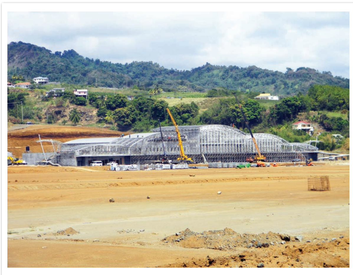
Photo 5.1: Construction Site - Argyle International Airport
