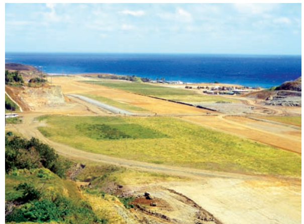
Photo 6.19: Argyle International Airport: Northern View of Runway Under Construction
