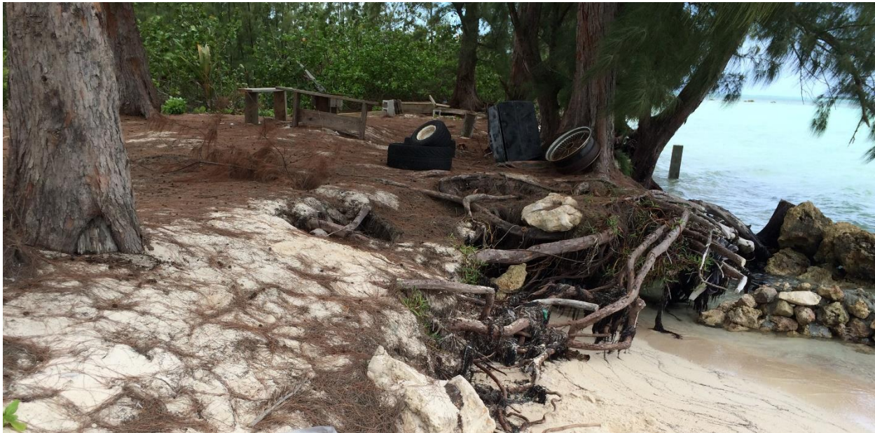
Picture 38: Coastal Erosion on Andros Island
