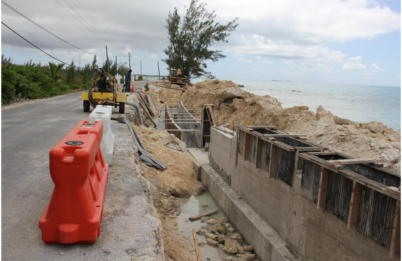
Picture 30: A New seawall being constructed on the Family Islands.
