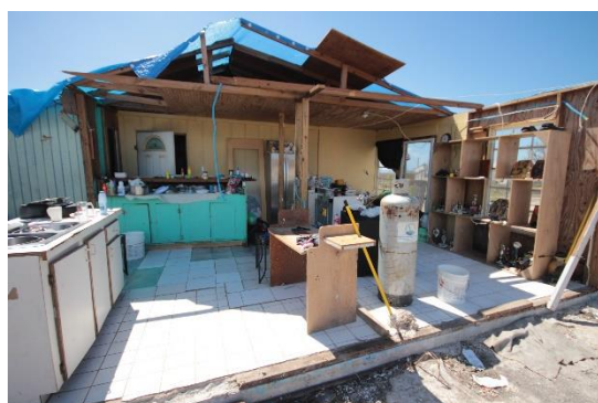
Picture 31: House destroyed by hurricane
