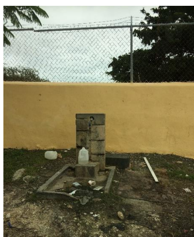
Picture 11: Typical standpipe found throughout The Bahamas to provide clean, safe potable water to residents who do not have access to piped water
