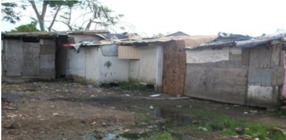
Picture 32: An informal settlement in New Providence. Photo Credit: D.E.H.S Shanty Town Project 2013
