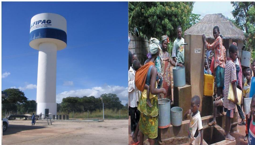
Figure 4.5 – Water tank and standpipe in Mozambique
