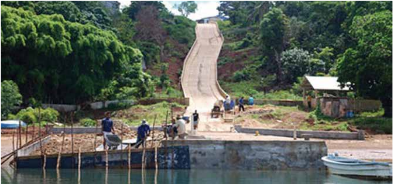
Figure 11: Road and jetty project at Hunga Island
