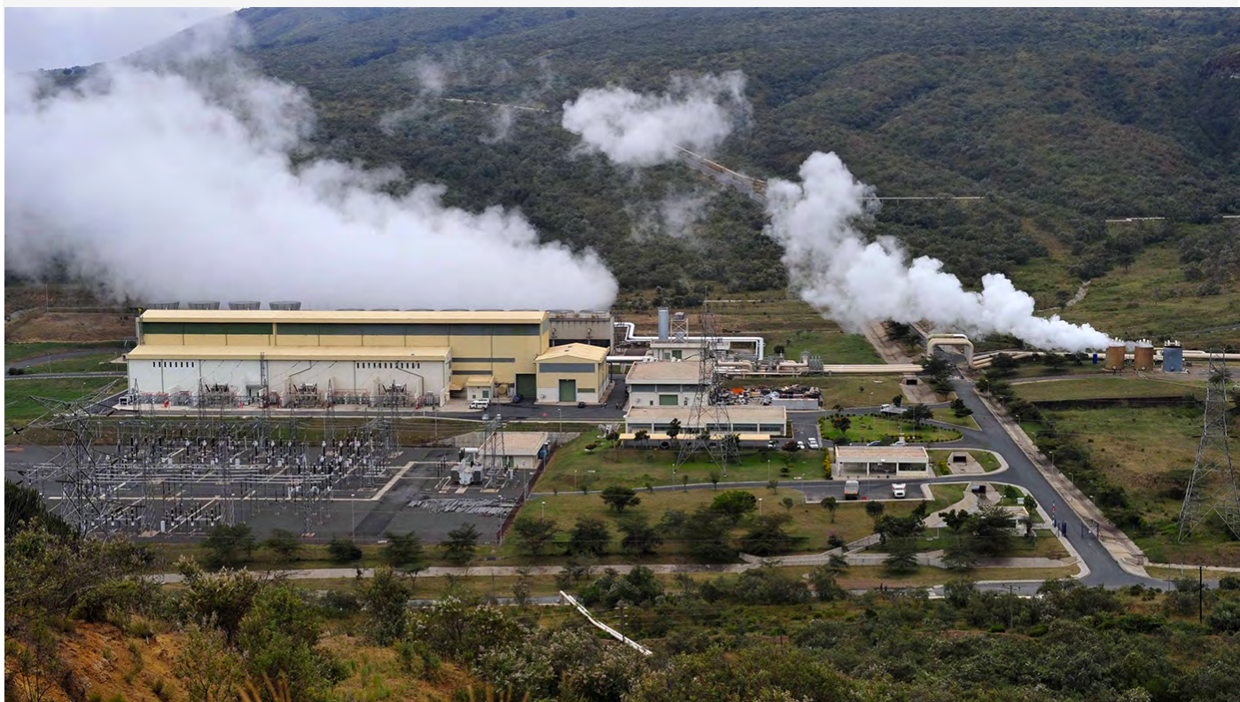
Olkaria Geothermal Power Station.
