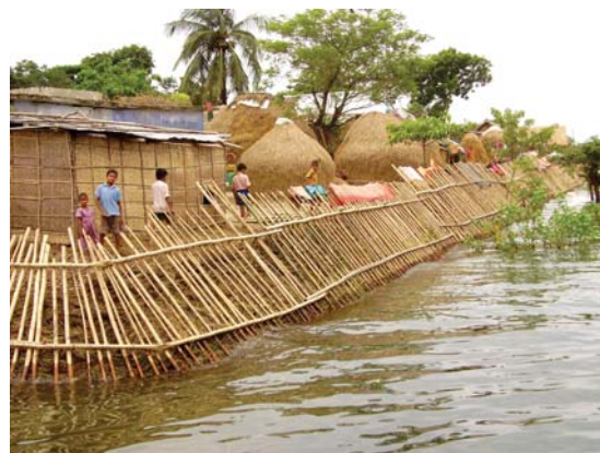
Community led initiatives-Protecting village from wave erosion, Sunamganj. Source: CDMP II
