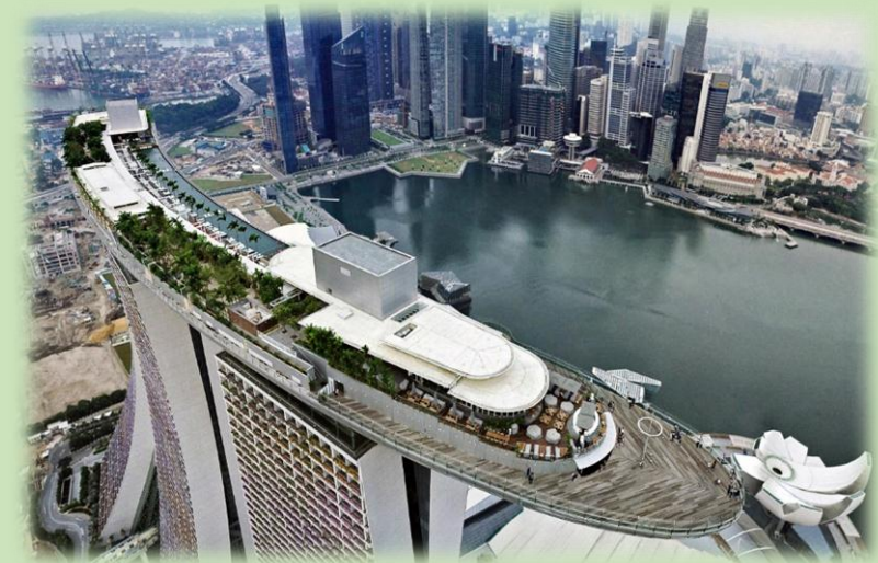
Rooftop park on the top of Marina Bay Sands
