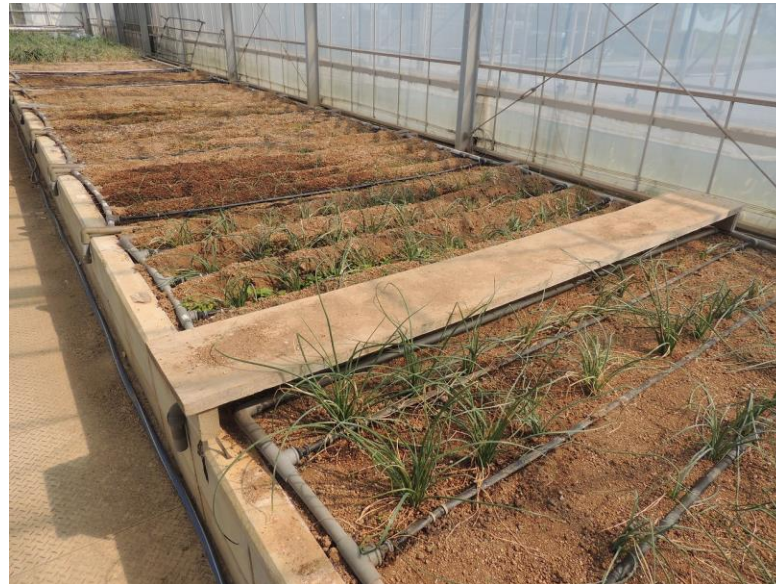
Cooling pipe system
