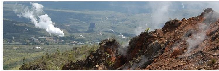
Photo of Geothermal wells at Olkaria by GDC
