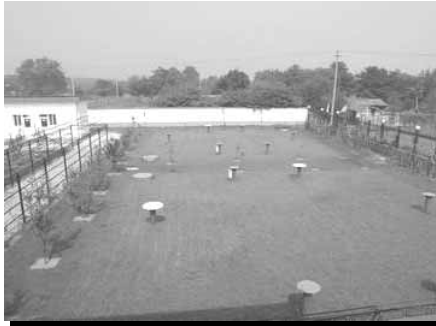
Water supply works
