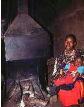
A hood over a fireplace
