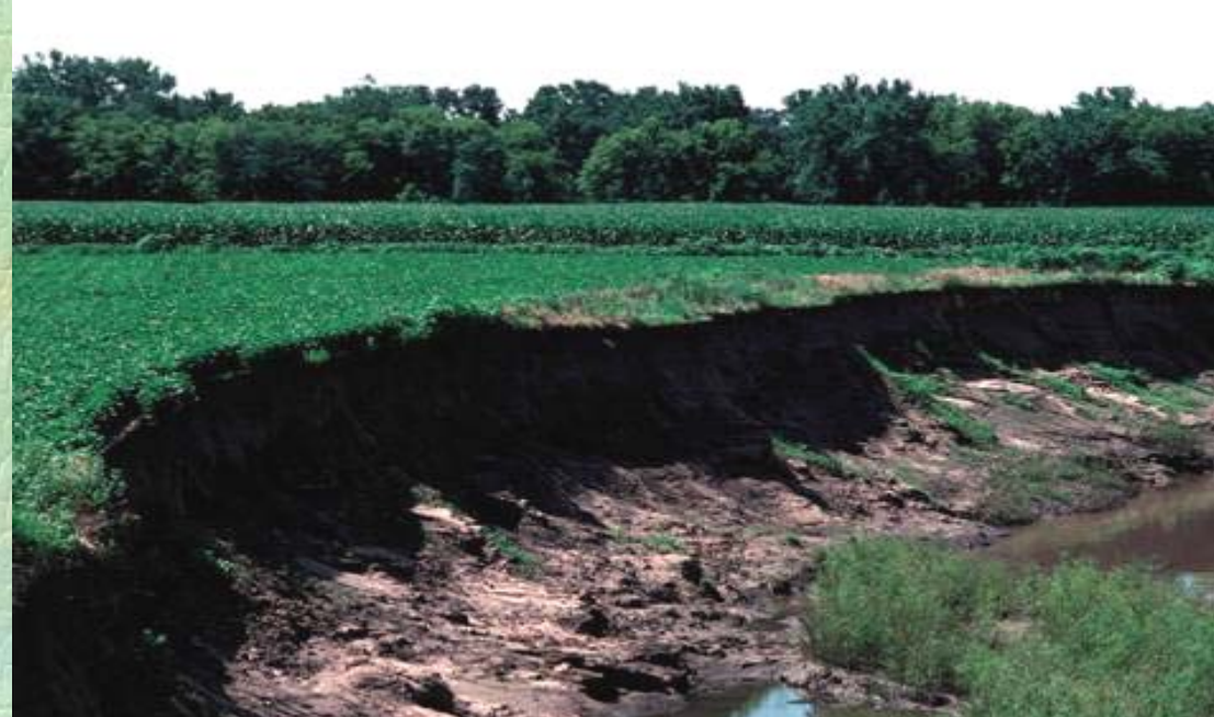
Bank Channel Erosion
