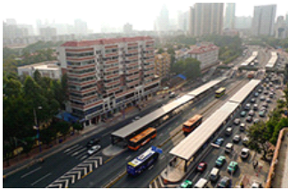
The longest Shidajida BRT station
