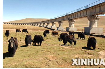
Elevated track & migration channel
