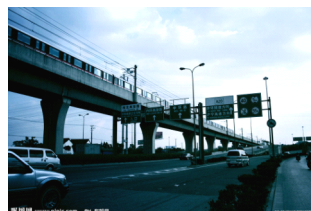
Rail on Overbridge
