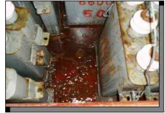
[Improper storage of PCB waste]
