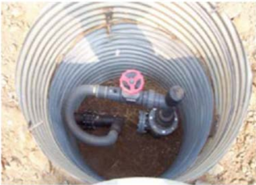
Landfill gas extraction well installation
