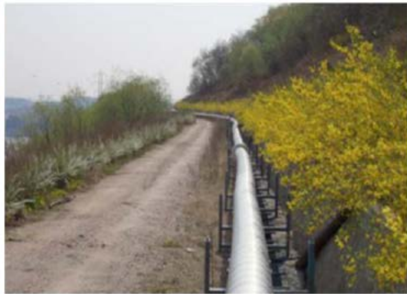
Landfill gas transport pipe being installed on slopes
