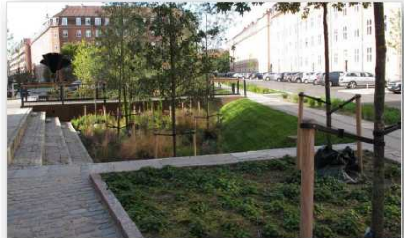
Storm water storage space at Tåsingeplads in Copenhagen, Denmark
