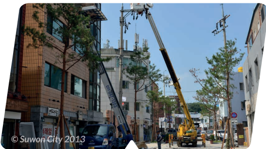
3. Removal of overhead utility poles to prepare for burying of cabling in August 2013
